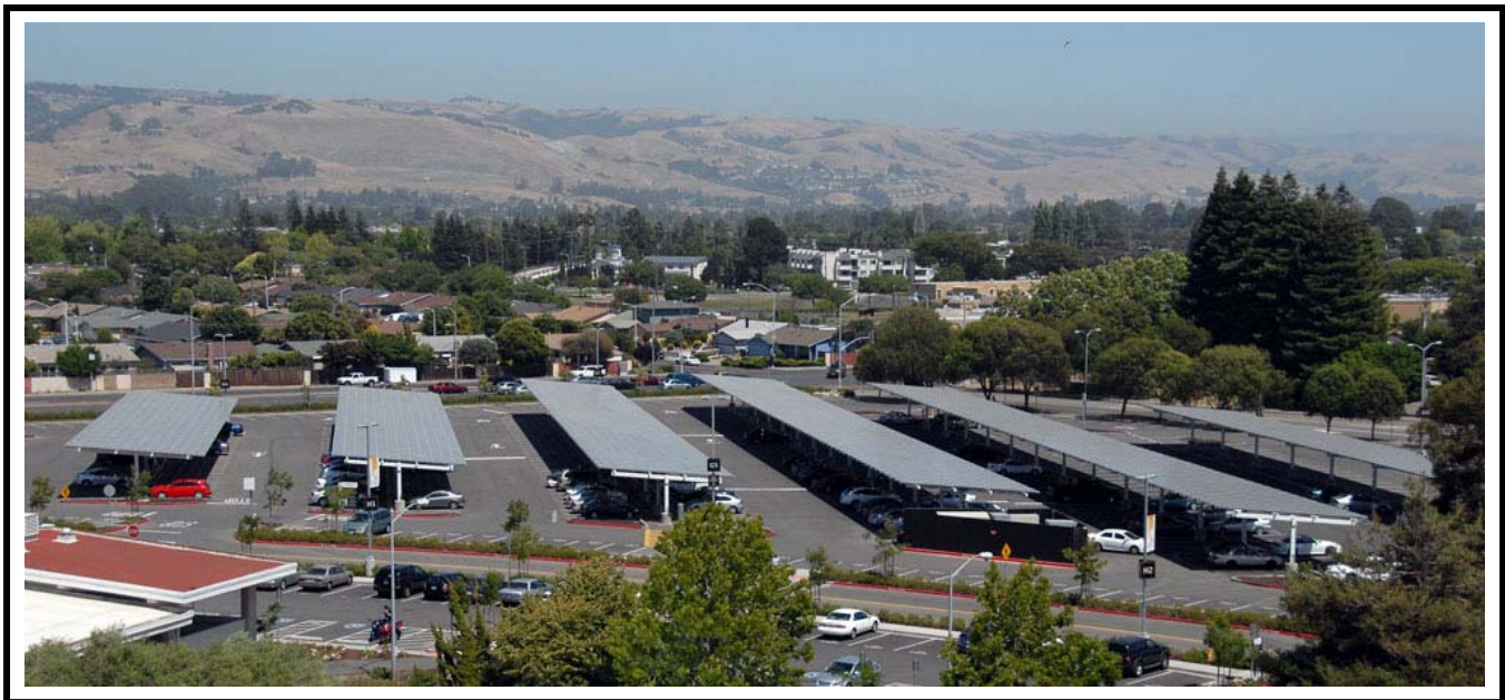
Lot G with Photovoltaic
